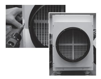
**Step 3:** Attach ducting as needed.
