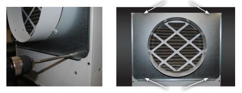
Note: 35" foam tape can be used to wrap around the duct collar to provide a seal between the duct collar and the duct plate (optional).
