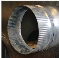
**Figure 2:** Install the 6" duct collar.
