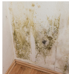
Mold growth on an interior wall. Over-cooling the space to control the humidity.
