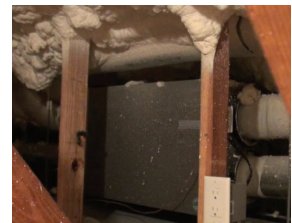
Energy Recovery Ventilator installed in the home.
