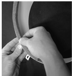
**Step 3:** Using the self-drilling screws and the hex or nut driver, attach each 10" collar to the dehumidifier by lining up the tabs on the collars to the pre-drilled holes in the cabinet around the supply / discharge on each side of the dehumidifier. Once in place, firmly tighten all four screws for each collar.
